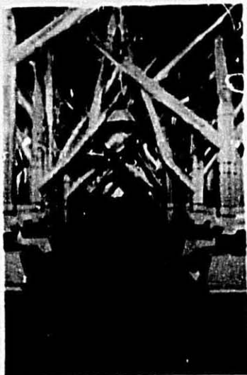
A forest of metal tubes brings air to the purifying operation.
